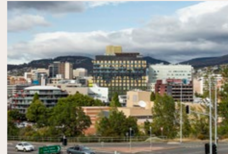
ROYAL HOBART HOSPITAL REDEVELOPMENT – LYONS WITH TERROIR
