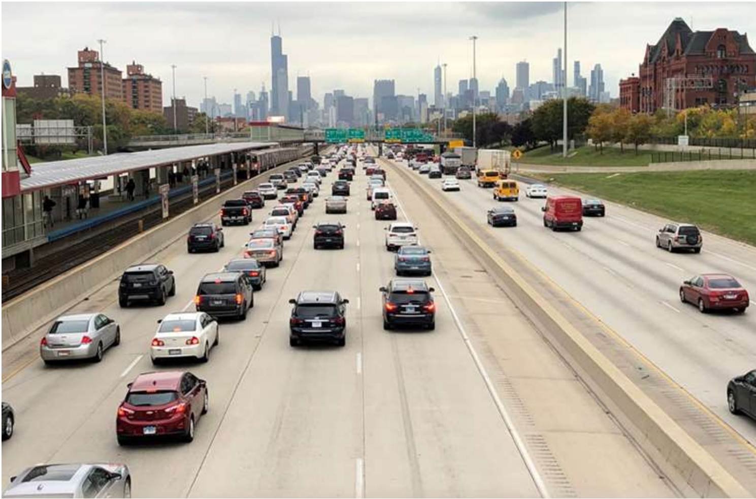
Dan Ryan Expressway + Sox 35 th Subway Station
