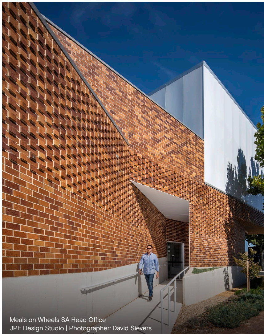
A person walking down a ramp of a brick building
