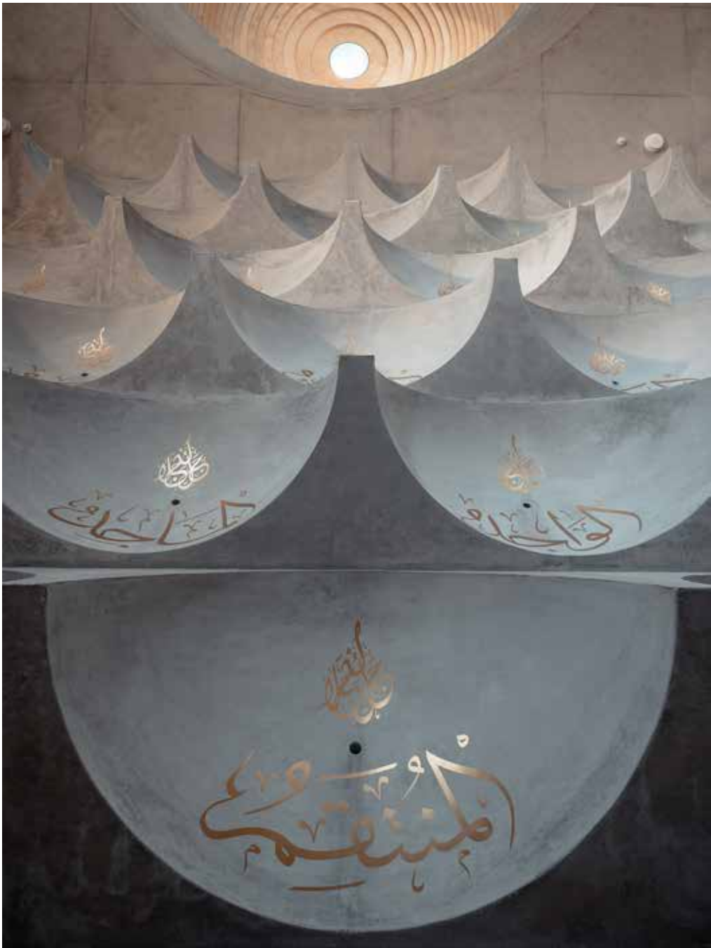
View of the concrete muqarnas domes with calligraphy depicting the 99 names of Allah and the timber-lined central dome with oculus at Punchbowl Mosque by Candalepas Associates Photo: Brett Boardman
