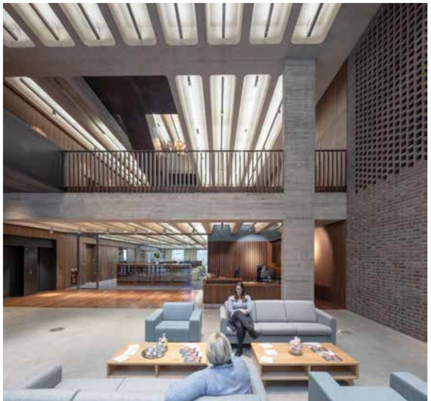
Environmental efficiency plays a key role in the design of Royal College of Pathologists building with exposed coffered concrete slabs used throughout the building to form part of the passive cooling strategy. By increasing the surface area of thermally active concrete, Bennetts Associates significantly improved the environmental efficiency of the building
