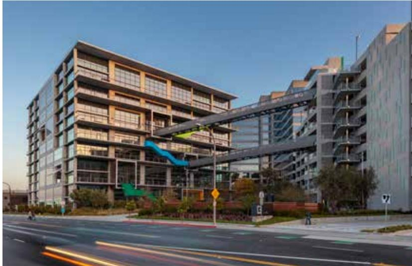
Dis-conditioning spaces by moving stairs outside relieves the need for heating and cooling them thus reducing operational energy. This move also creates a positive experience for building occupants by giving individual front doors for tenants occupying upper floors of office buildings. Photo courtesy Gensler
