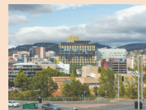
Royal Hobart Hospital Redevelopment, Lyons with Terroir
