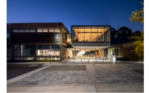
EDUCATIONAL ARCHITECTURE JOHNS XXIII COLLEGE, ANU COX ARCHITECTURE BUILDER: CAPCORP GROUP PHOTOGRAPHER: JAKUB BESEDA
