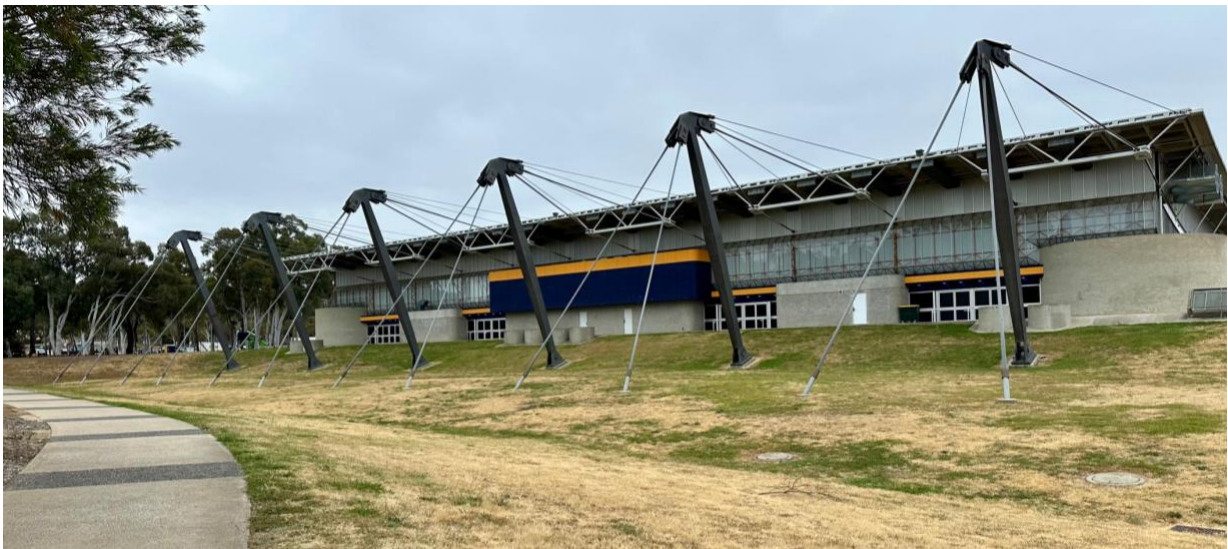
East side of AIS Arena (2025)
