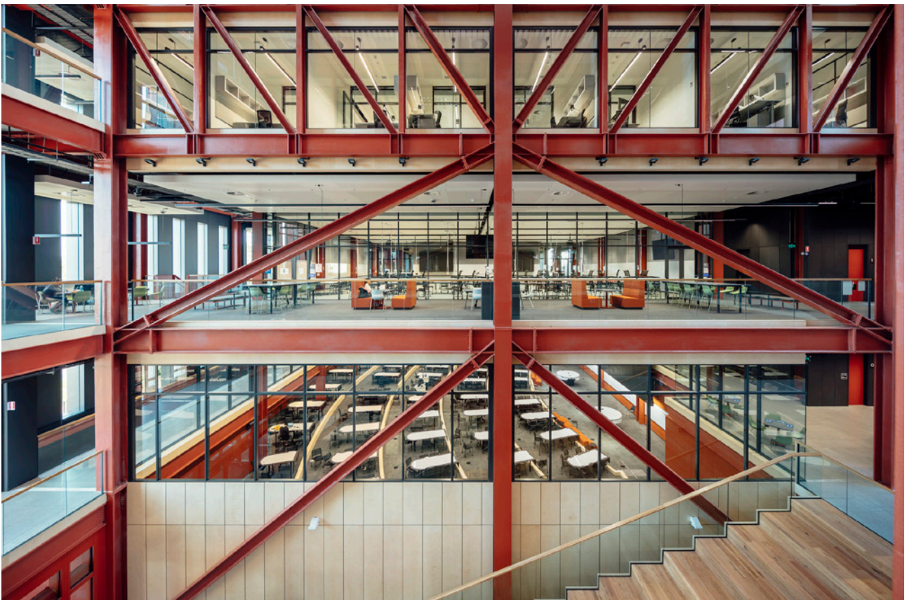
Monash Woodside Building for Technology and Design | Grimshaw in collaboration with Monash University | Photographer: Rory Gardiner
