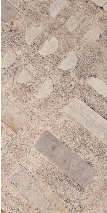
Reuse, taking excavated artefact's from the site, slicing them and laying into a large public space for story telling and pattern.
