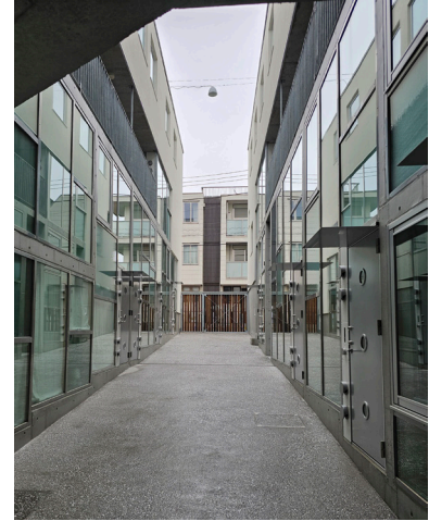
Figure 32. Open, semi-public space, Jingumae Void Infrastructure, 2024, Shibuya-ku, AWN.
