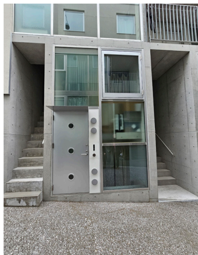
Figure 39. Threshold to maisonette, Jingumae Void Infrastructure.
