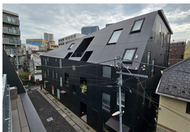
Figure 29. View of Kif from 'front yard' of upper-level apartments in Kif Annex.
