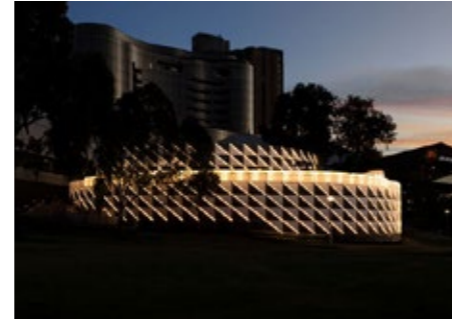
CITY OF ADELAIDE PRIZE ADELAIDE FESTIVAL PAVILION CO-AP ARCHITECTS PHOTOGRAPHER: ROSS HONEYSETT
