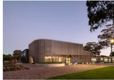
EDUCATIONAL ARCHITECTURE HAMILTON SECONDARY COLLEGE PERFORMING ARTS CENTRE TOTALSPACE DESIGN PHOTOGRAPHER: COREY ROBERTS
