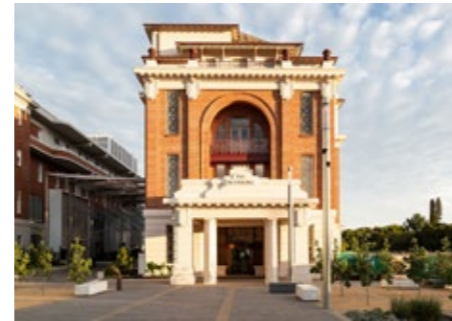
CITY OF ADELAIDE PRIZE BICE BUILDING REFURBISHMENT HASSELL, PURCELL AND BAUKULTUR PHOTOGRAPHER: RAPHAEL CHRISTINAT (BAUKULTUR)
