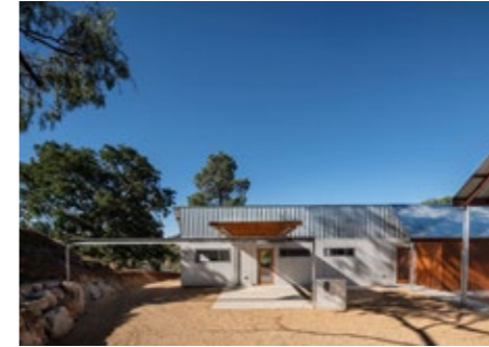
RESIDENTIAL ARCHITECTURE – MULTIPLE HOUSING ANGASTON HILL TAYLOR BUCHTMANN ARCHITECTURE PHOTOGRAPHER: PETER BARNES
