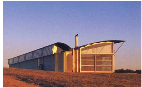
View from southeast (Photo: Anthony Browell from M Gusheh, T Heneghan, et al. The Architecture of Glenn Murcutt , 2008)
