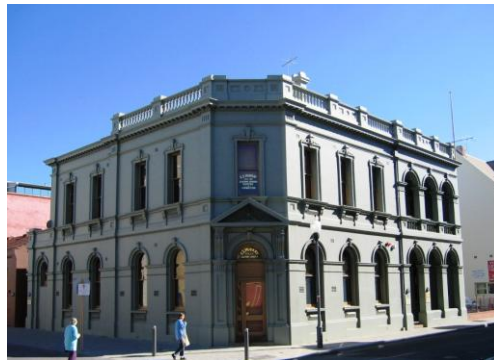
Union Bank of 1889 on the corner of High and Cliff Streets, Fremantle (John Taylor, July 2008)
