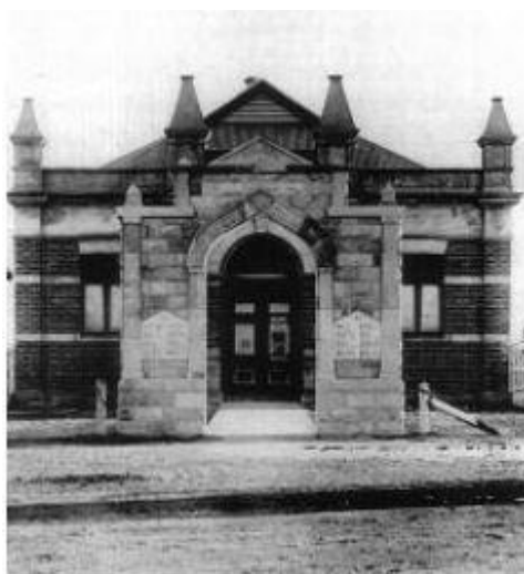
Downes designed this Donnybrook stone war memorial of 1921, shown in its original position outside Canning Town Hall (Stephens, John, 'Community meaning and heritage of Western Australian war memorials', Fig.1 - with acknowledgement to Canning Districts Historical Society)
