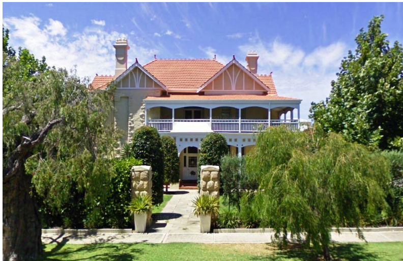
58 Leake Street, Peppermint Grove (Google 2012)
