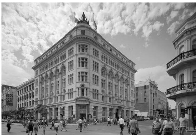
AMP Building, cnr St George's Terrace & William Street, Perth, shortly before its demolition in 1972 (Fritz Kos SLWA 341133PD)
