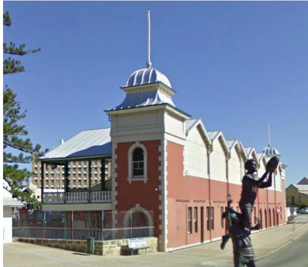
Fremantle Oval Grandstand, Parry Street Fremantle 1897 (Google 2013)
