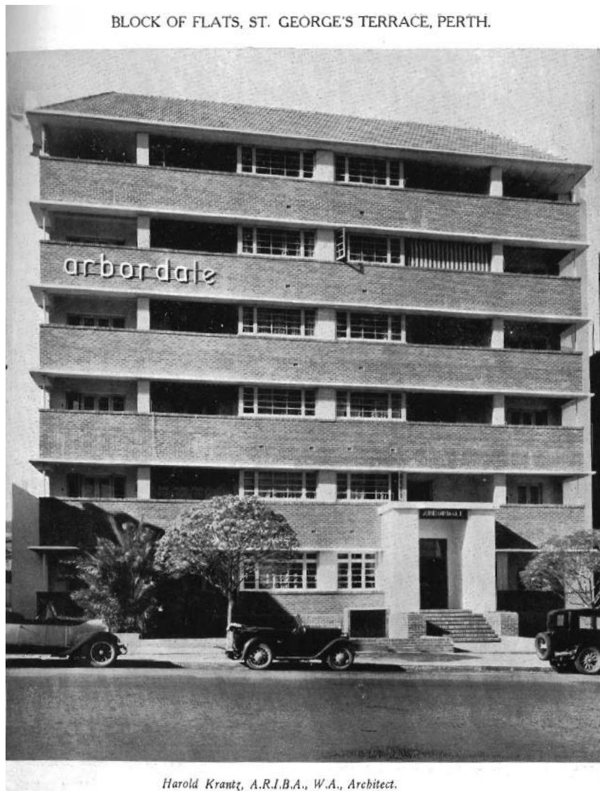
'Arbordale' Flats, St George's Terrace Perth have been demolished ( The Architect , Vol 1, No 11, December 1939, p.21)
