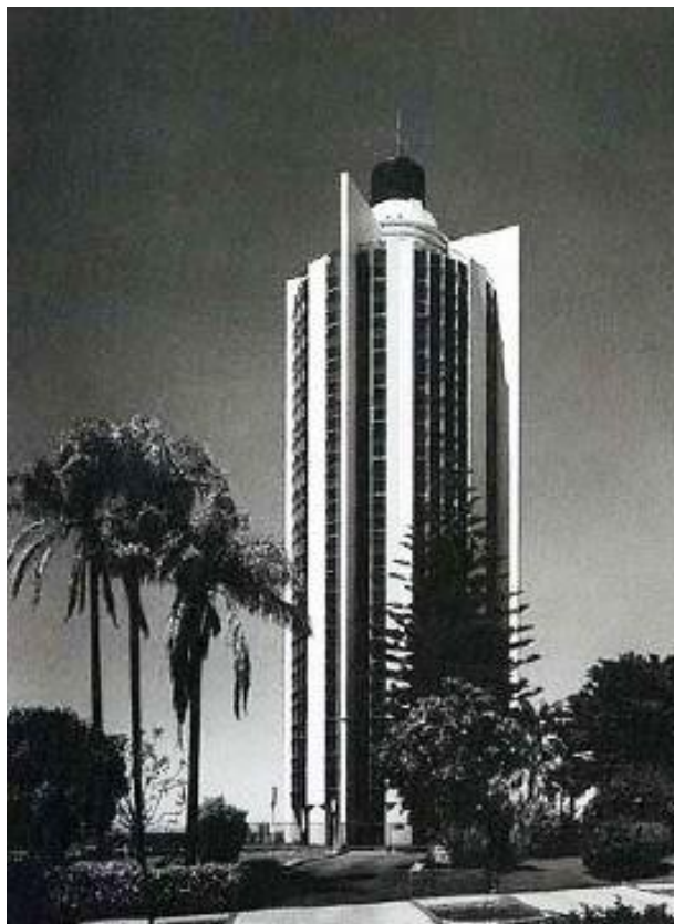
Mount Eliza Apartments of 1964, West Perth effectively marked the change in generation from Harold Krantz to son David ( http://watvhistory.com/2012/06/remembering-dorothy-krantz/ ).
