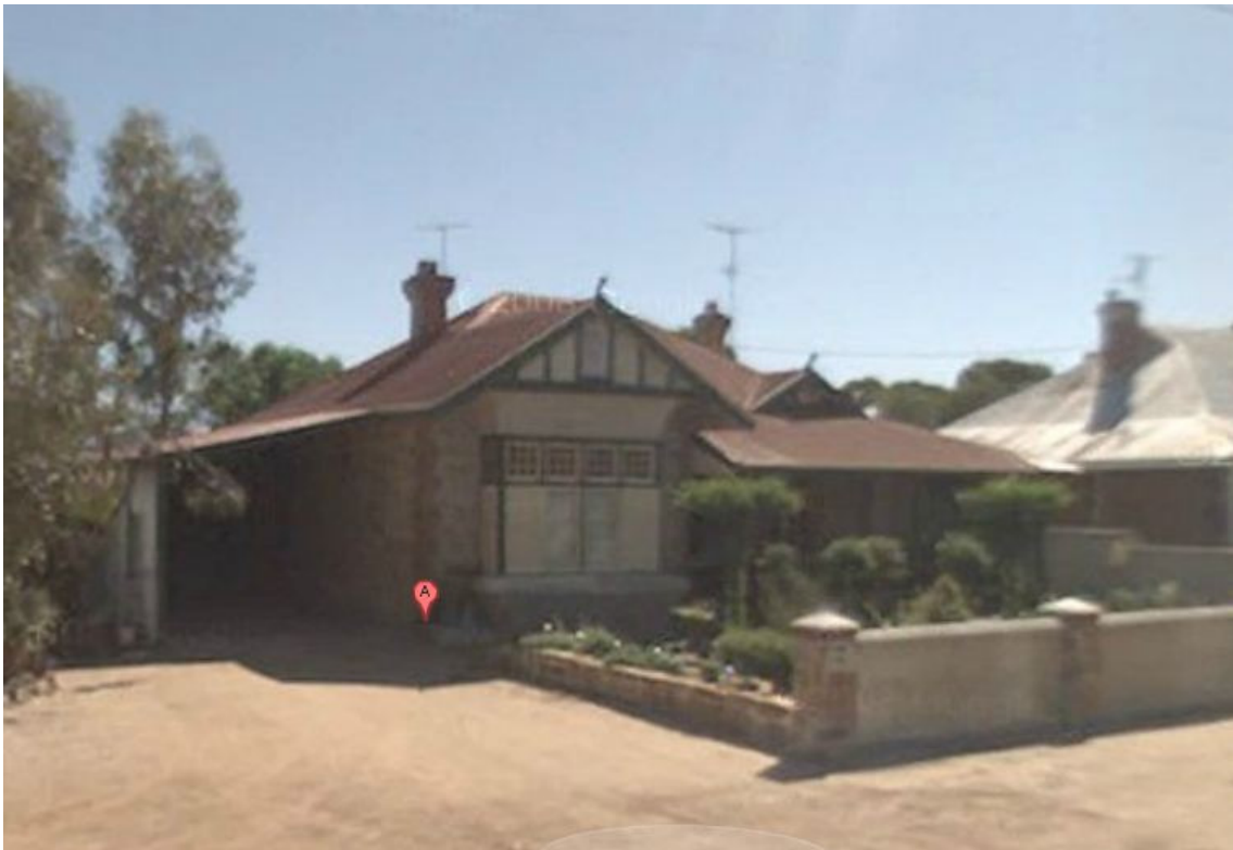
1913 Anglican Rectory (fmr), 61 James Street, Kellerberrin (Google 2012).
