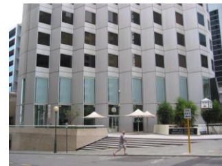
Ground level of Allendale Square from the north-east (Katrina Chisholm, 2011)
